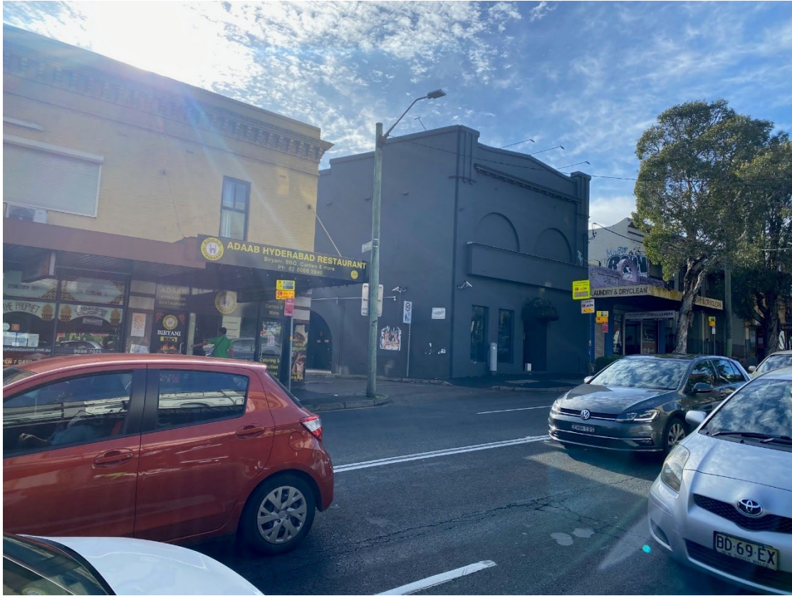
adjoining development on Cleveland Street – to east
